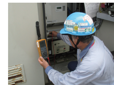
検電作業 Electricity detection
