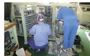
最新機種への換装工事 Conversion to the latest equipment
