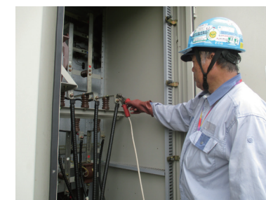
放電作業 Discharging job
