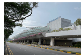
Changi Airport T2 LT REPLACEMENT (2022年竣工)
