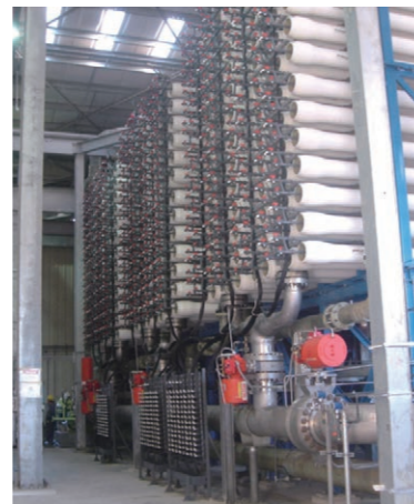
独自の熱誘起相分離法による強靱さと精密細孔を併せ持つPVDF中空糸膜 PVDF hollow fiber membranes featuring both toughness and a precise pore structure due to our unique thermally induced phase separation method
