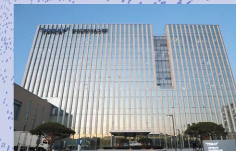
Toray Advanced Material Korea Inc. <TAK>
